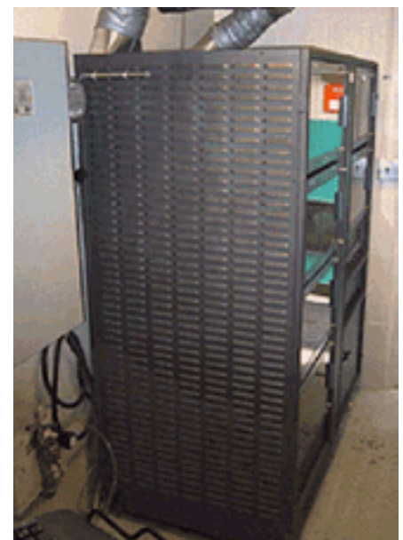
This 3kW fuel cell has been tested in a pilot application for the military since 2002
