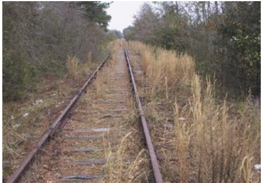
This abandoned rail line along Spruill Avenue that could become a recreational trail.
