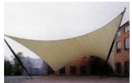
An example of a performance space transforming an industrial area.
