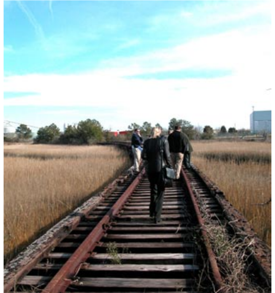
Existing conditions at the elevated rail line looking east.
