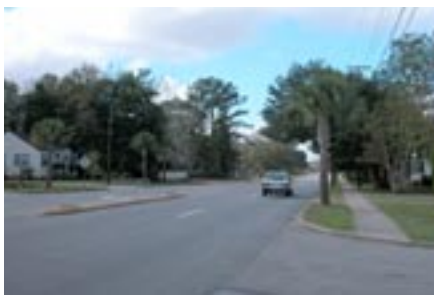
Image looking down Montague Avenue
