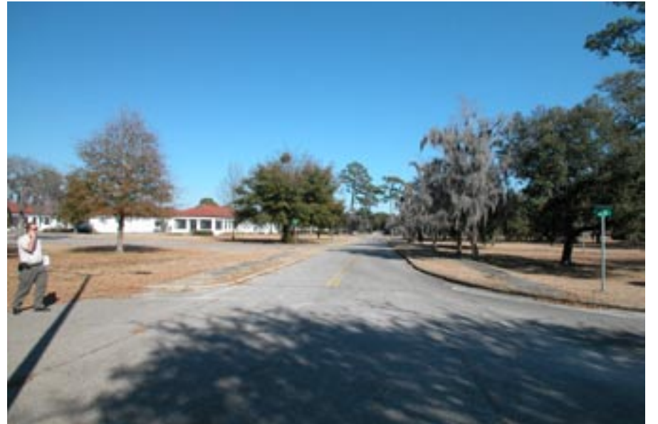
Existing Naval Base Conditions
