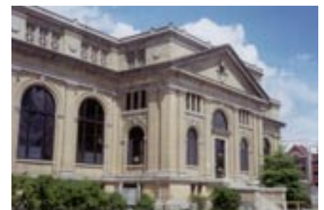
The old Power House in the beaux arts tradition.
