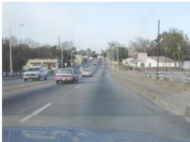
Existing conditions of Cosgrove looking to the proposed River Center at Noisette
