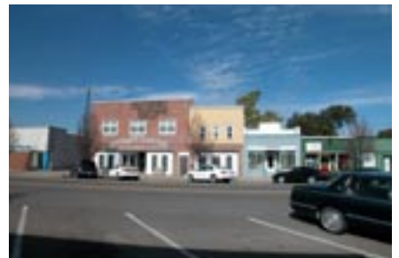
Existing East Montague storefronts with on-street angled parking.
