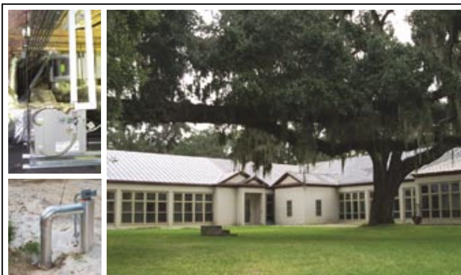
Mepkin Abbey Geothermal heat pump system designed by Burt Hill
