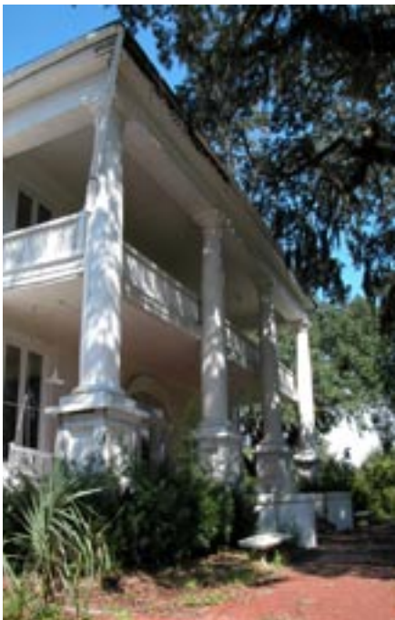
Important heritage sites will remain and flourish, through which a new image will result, unlike any other.
