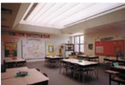
High quality daylight enters classrooms through windows and roof monitors. Combined with the light-colored interior finishes, this reduces the amount of energy expended to light each classroom.
