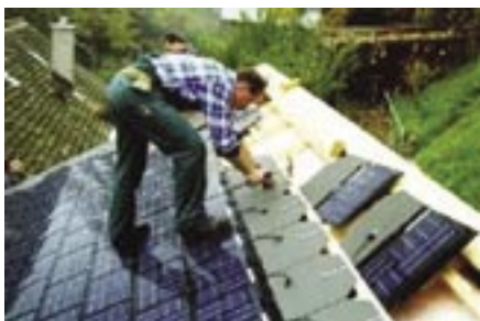
BIPVs are available in units that can be installed using conventional construction techniques
