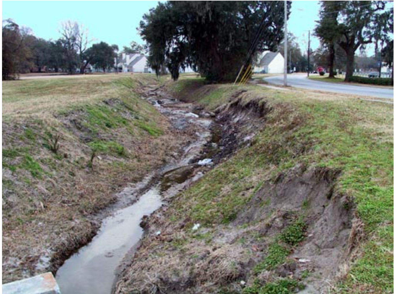
This stream in the Century Oaks area was turned into a drainage ditch to provide conveyance by incising its channel and disconnecting it from the floodplain. The result is unstable eroded slopes and increased downstream sediment loads. Establishment of natural stream geometry and connection to a floodplain would help restore this ditch to a stream.
