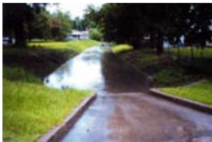
The absence of source management has resulted in this channel conveying considerable water during a relatively minor storm event.
