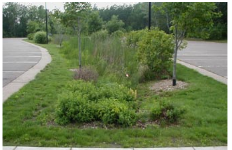
Bioswale in parking lot application
