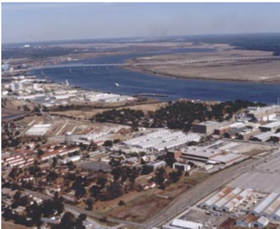
Aerial view of the former Charleston Naval Base, the location of the proposed River Center at Noisette.
