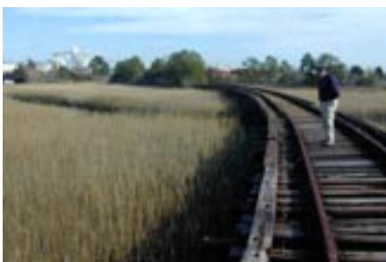
Elevated line on east end will remain as industrial artifact
