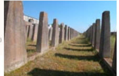
Cribbing once used for large steel plate stands in the Interim Arts Park area.
