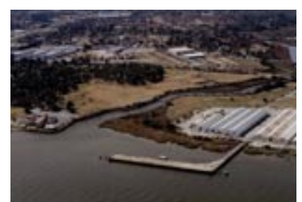
Pier Alpha at the junction of Noiset Creek and the Cooper River
