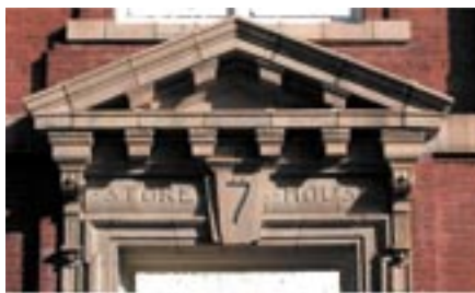
Building 7 of Storehouse Row
