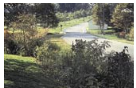
Example of an existing small-scale vegetated bioswale. As the swale gets larger, it would turn into a forested corridor swale, with an engineered system of pools and riffles in the channel, vegetatively reinforced side slopes, and an appropriate upland buffer.
