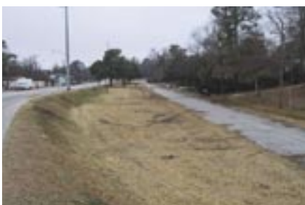
Low-lying area, such as this one off Spruill Avenue, have the potential to serve as vegetated infiltration retention areas and eliminate considerable runoff volume, while trimming peak runoff discharge rates downstream.
