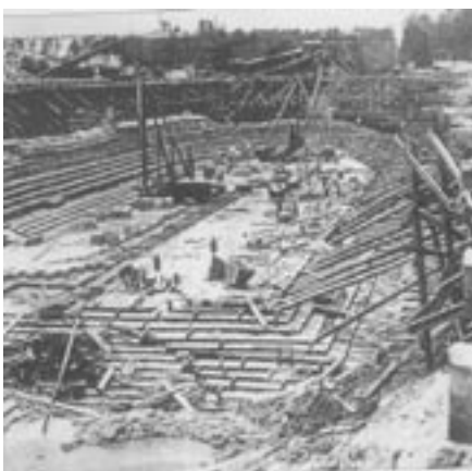
Charleston Naval Base dry dock
