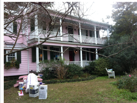
Above: This home built in 1880 received a energy retrofit that included air sealing, insulation upgrades and a new efficient HVAC system.
